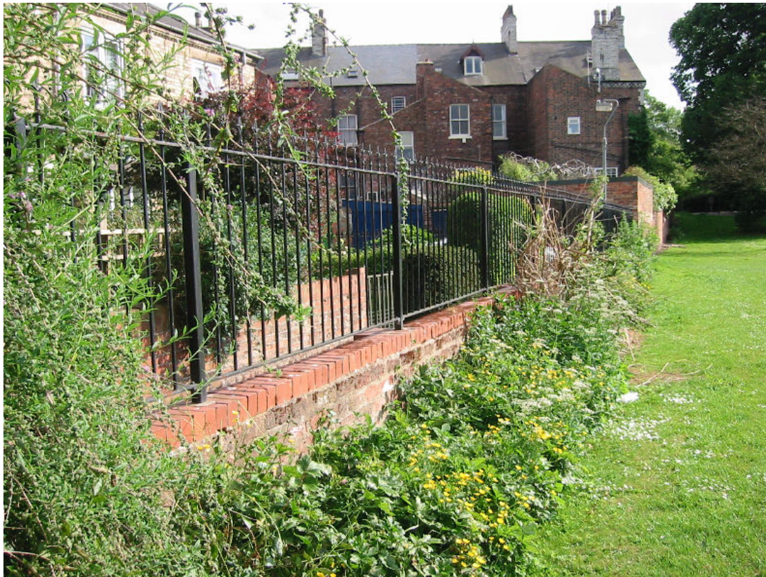
c) Boundary wall and railings – looking in a southwesterly direction towards the back of properties on Scarcroft Road.
